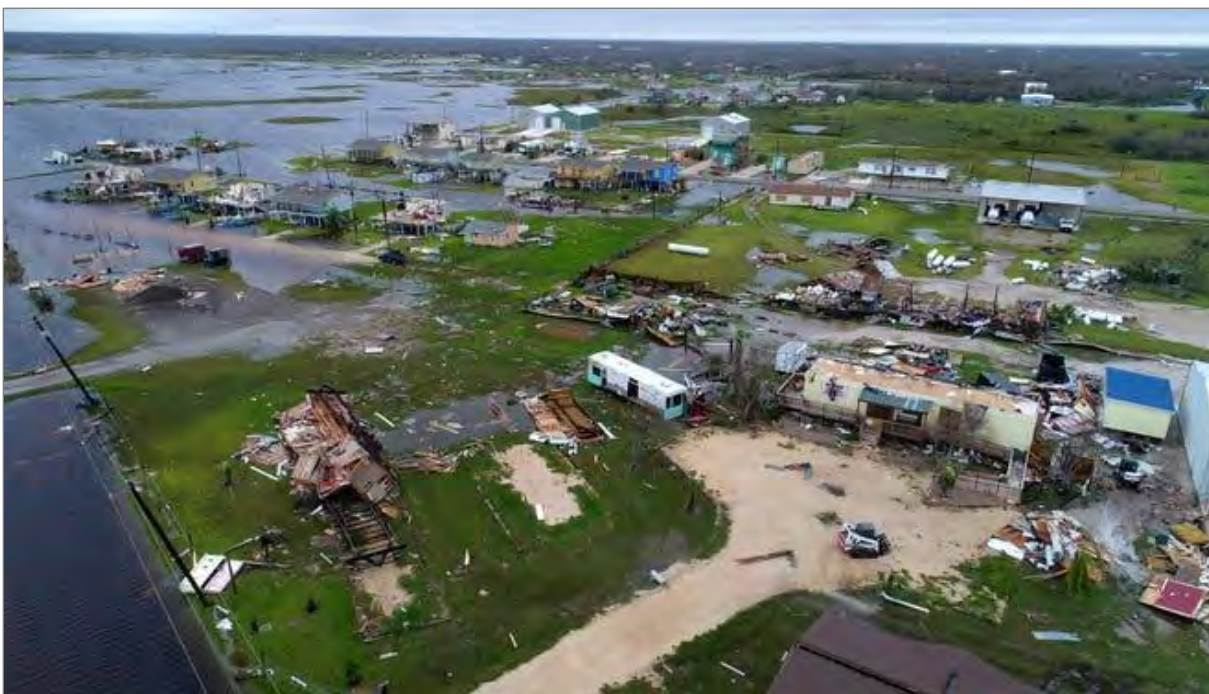
Figure 11-1. Aerial Footage of Harvey Damage in the City of Rockport 5
